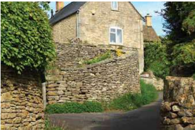
Stone boundary walls provide sense of enclosure.
